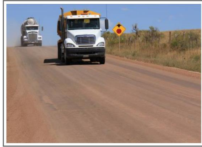
Stable fines preservation on a treated road
